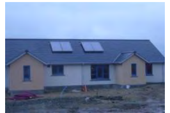
18 Units at Bridge Cottages Stornoway
