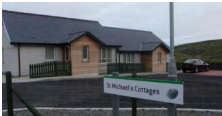
4 Units at St Michael's Cottages, Barra
