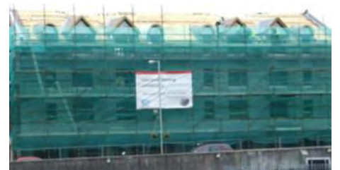
12 Units at Smith's Shoe Shop, (Ardanmhor Court) Stornoway
