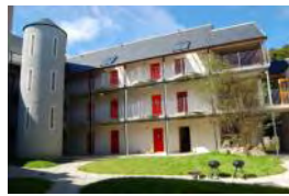
8 Units at the Bridge, Stornoway, Lewis
